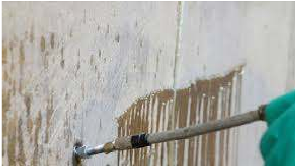
INJECTION GROUTING
