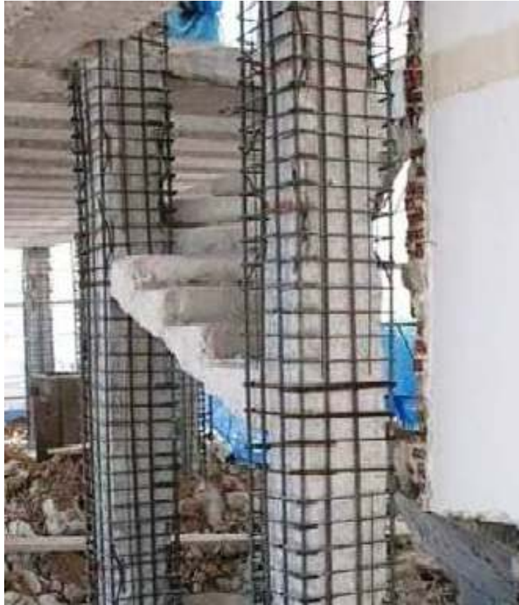
RCC JACKETING OF COLUMNS (Refer Item no. 8 in S.O.R.)
